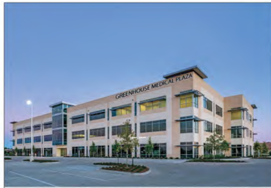
MRI GREENHOUSE Houston, Texas
